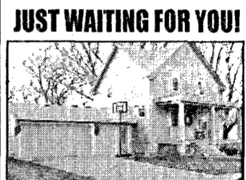
404 Elm, Laurel 3 bedroom, with new furnace, roof and windows. All appliances included.
