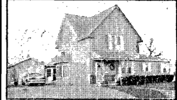
504 Oak, Laurel Ready to move into! Nice 2 story with fireplace.
